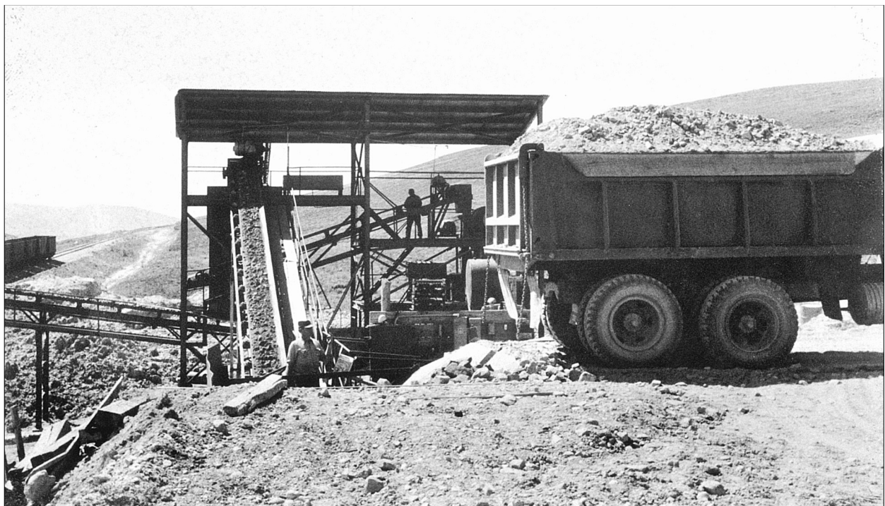
Figure 126. Loading Centennial Mine phosphate ore at Monida, Montana, September 23, 1957. BLM file photo.
